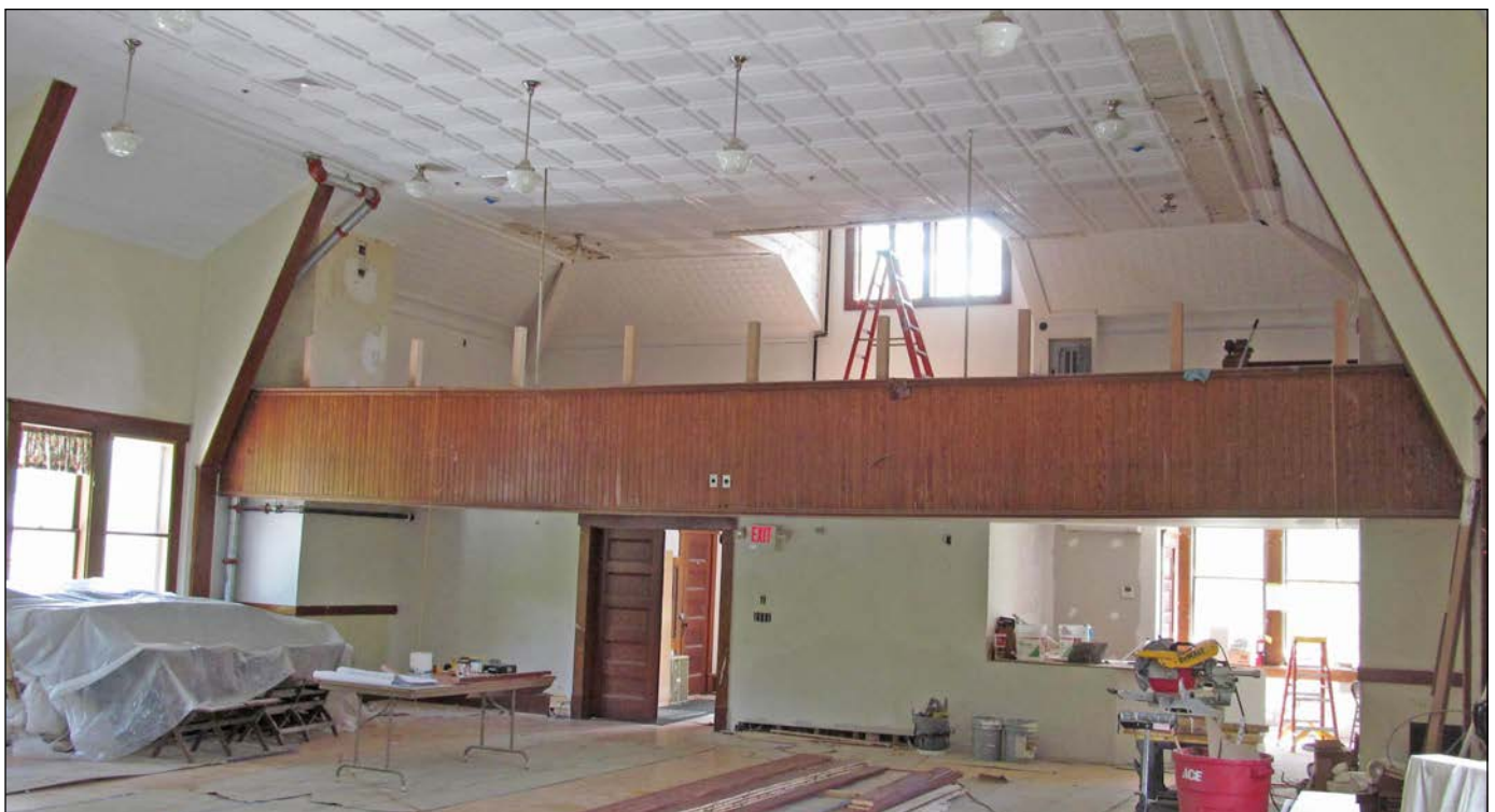
Renovation of the Fairlee Town Hall Auditorium
