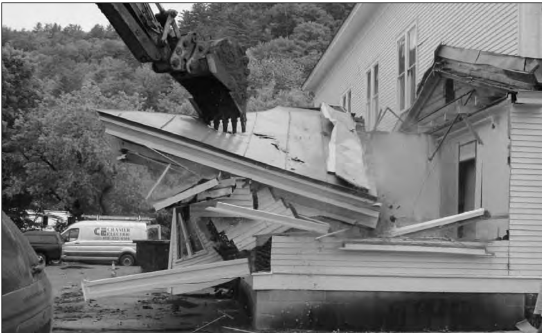
1950 addition removed May 31, 2017 for the new ADA addition
