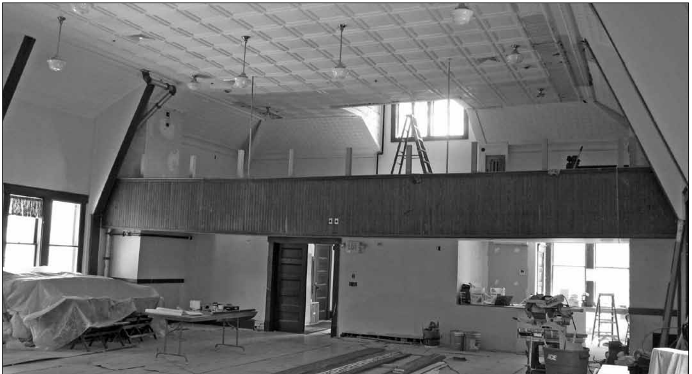
Renovation of the Fairlee Town Hall Auditorium
